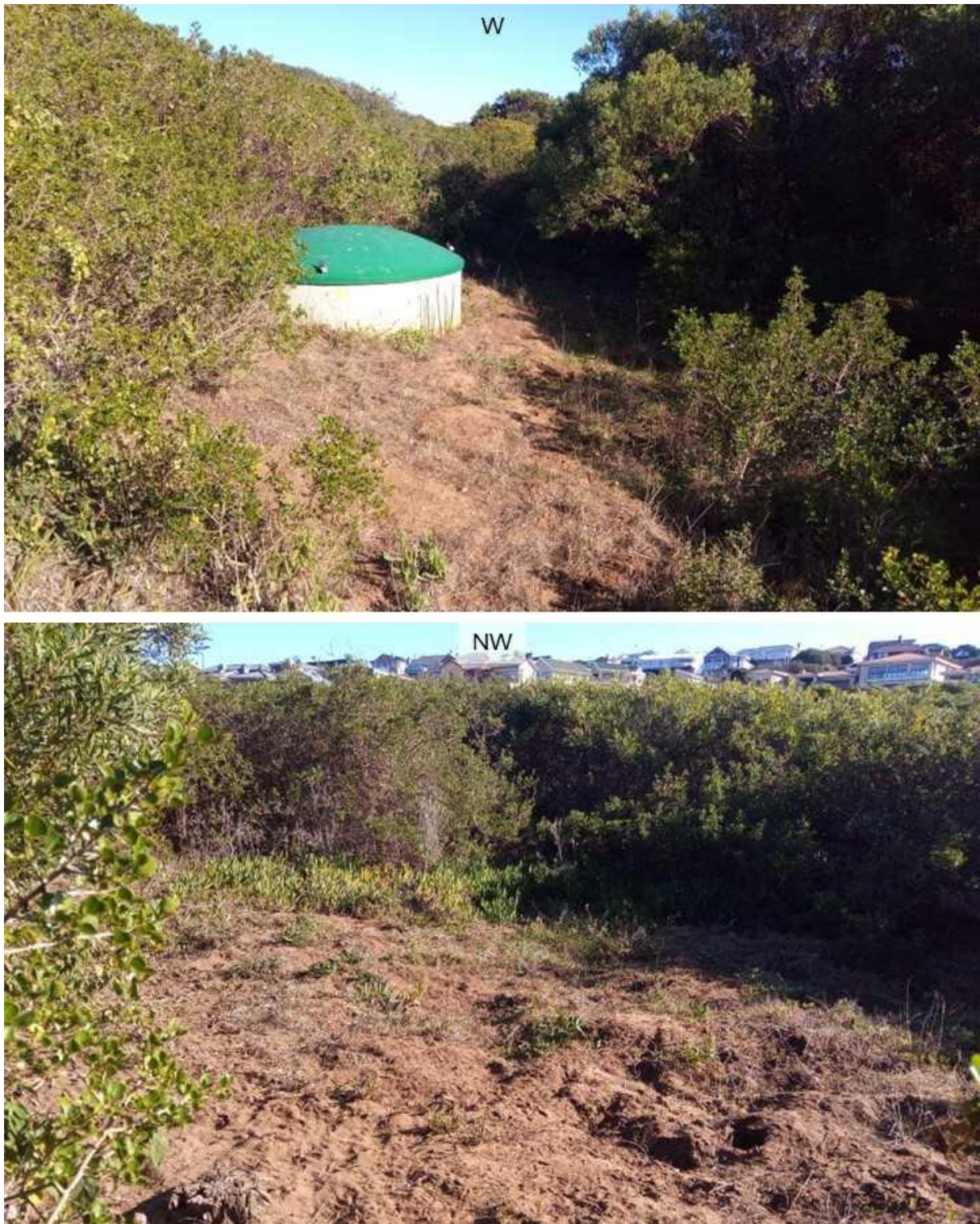
Figure 12. Examples of the receiving environment showing existing bulk service infrastructure, vegetation cover, exposed surfaces and mole heaps.
