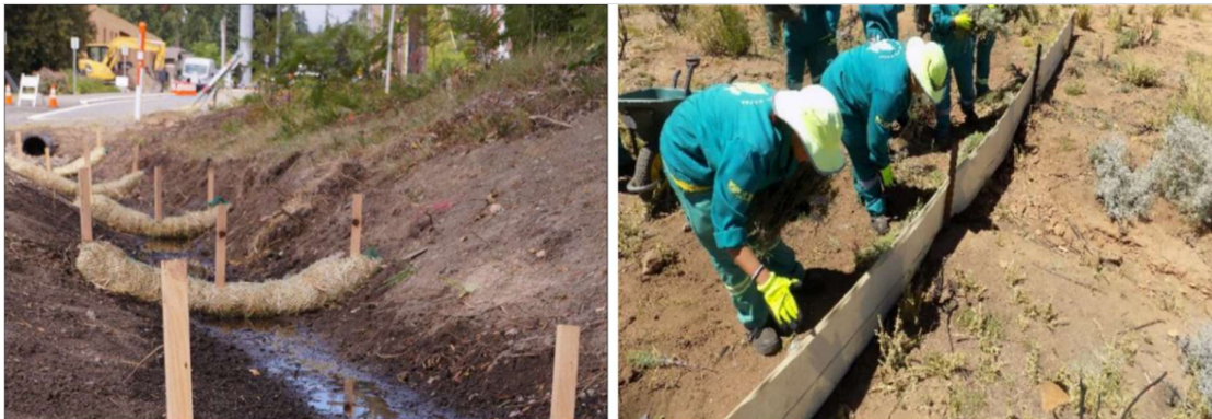
Figure 21. Examples of silt socks (left) and a silt fence (right) placed perpendicular to the flow of water. These methods reduce the force of water flow, erosion and can prevent unwanted sedimentation at the site.
