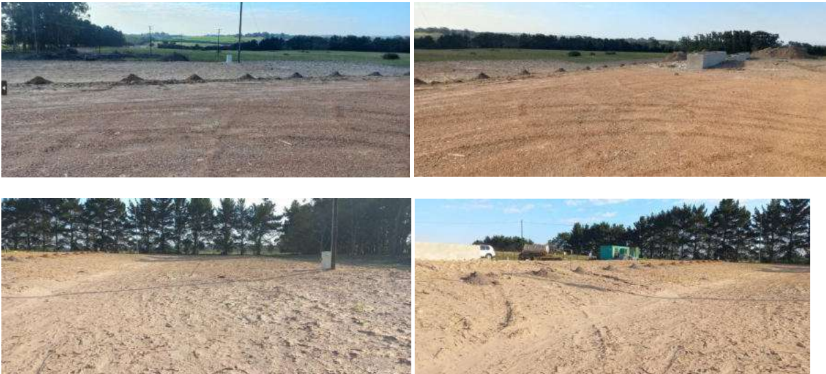
Figure 22: Photos indicating the construction of the aquaponics and fish farming facility.
