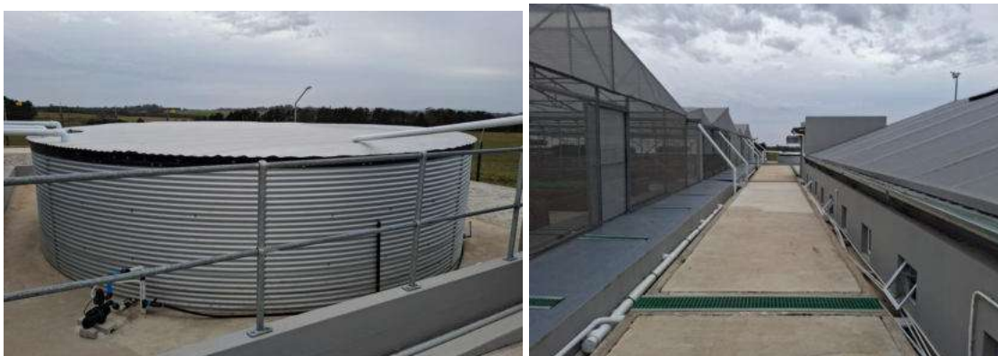
Figure 11: Recycled water in storage dam. All runoff from the facility is also captured and used in the system. No stormwater or nutrient rich water enters the natural environment outside of the facility.
