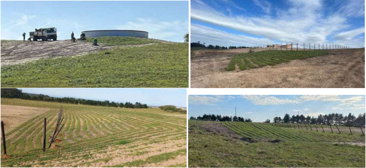
Figure 20: Areas being rehabilitated that were disturbed outside of the permanent development footprint.
