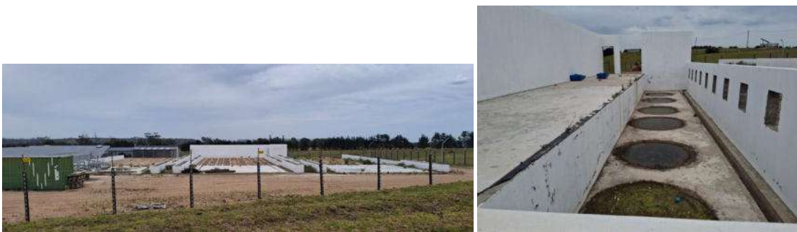
Figure 15: Phase 2 of grow houses and fish tank house half completed and not yet operational.
