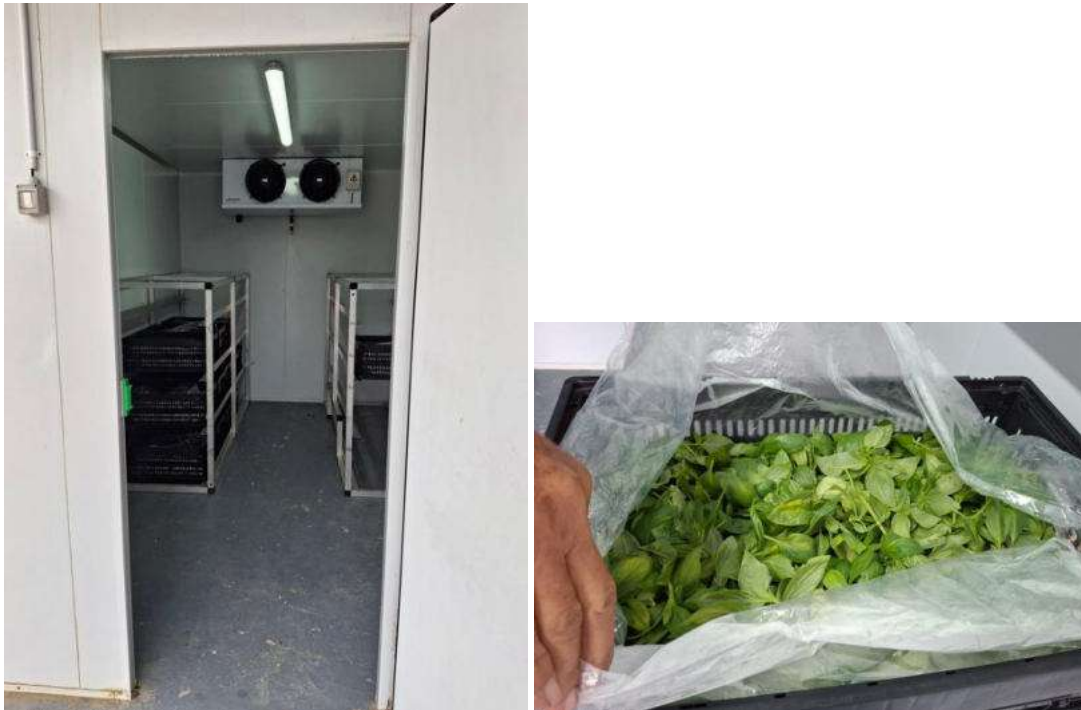
Figure 13: Fresh produce stored in the cooling facility ready for market delivery.
