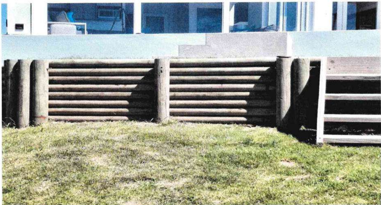
Picture 6: Showing the extension of the footprint of the house to the boundary of Erf 2520 with the stabilised embankment onto Erf 2514 which belongs to the Otters Landing Homeowners Association.
