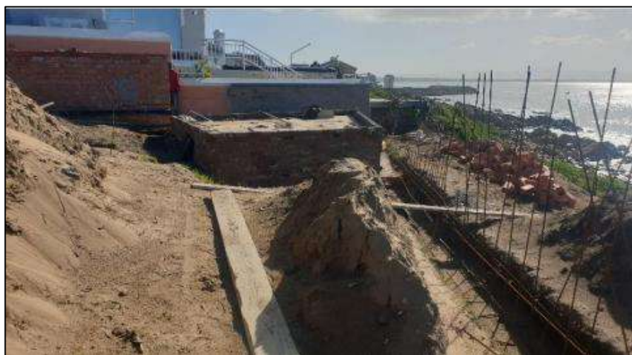
FIGURE 2: EXCAVATION ON SITE
