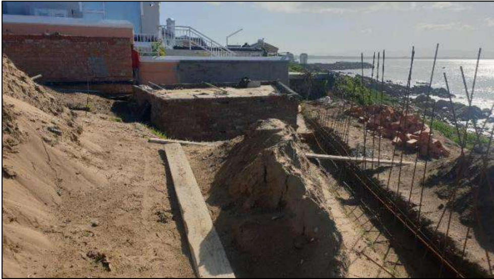
Figure 5: Excavations during construction phase on site
