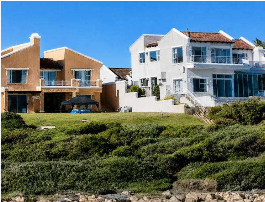
Figure 10: Previous house prior to demolition. Notice the grass area part of Otters Landing Open Space and the area beyond where the cement bench is situated, was there prior to the new construction.
