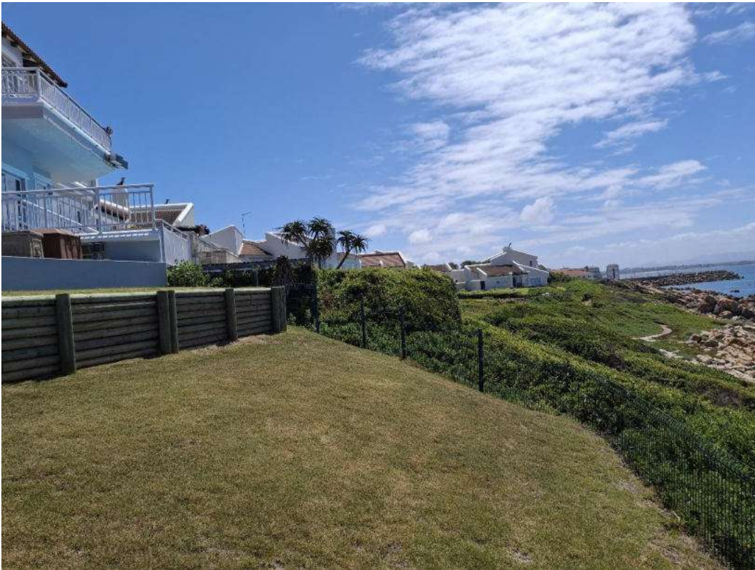
Figure 13: The area below the slope below the terrace will be rehabilitated
