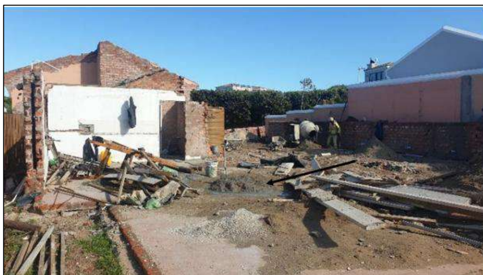
FIGURE 3: CEMENT MIXING TAKING PLACE ON FOUNDATION OF THE ORIGINAL HOUSE
