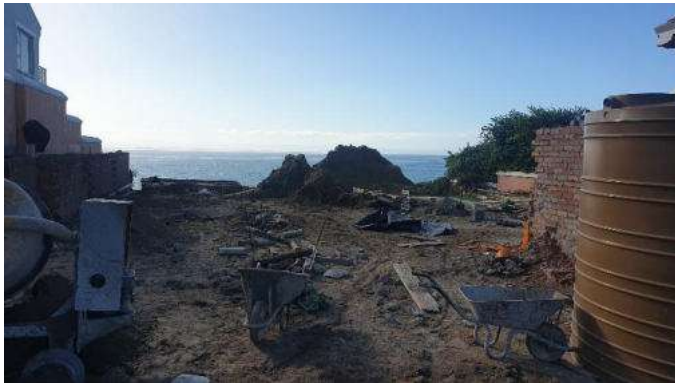
General site view from inland
