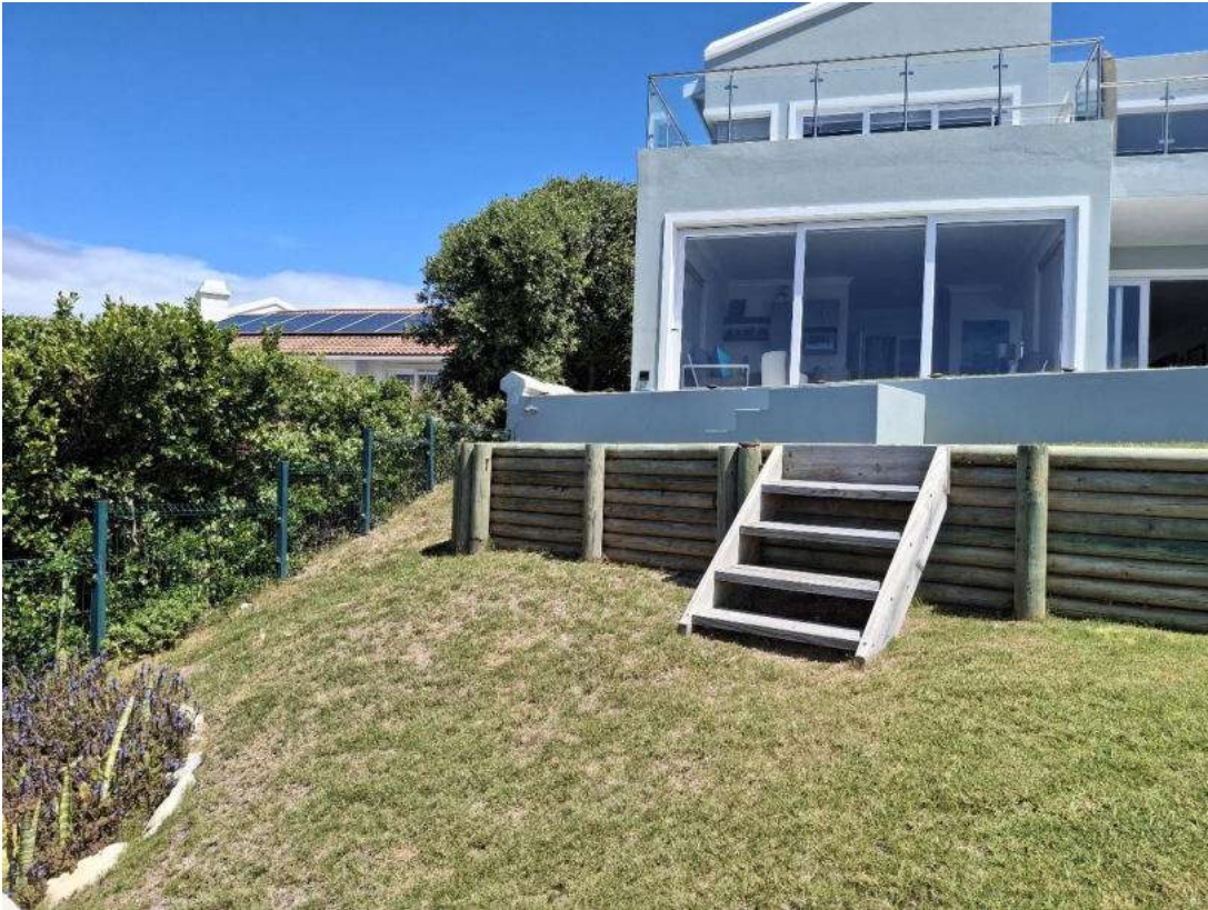
Figure 12: The area above the stabilised terrace forms part of the Otters Landing Homeowners Association private open space. The slope below the terrace will be rehabilitated with indigenous dune vegetation in accordance with the Environmental Management Programme (EMPr).
