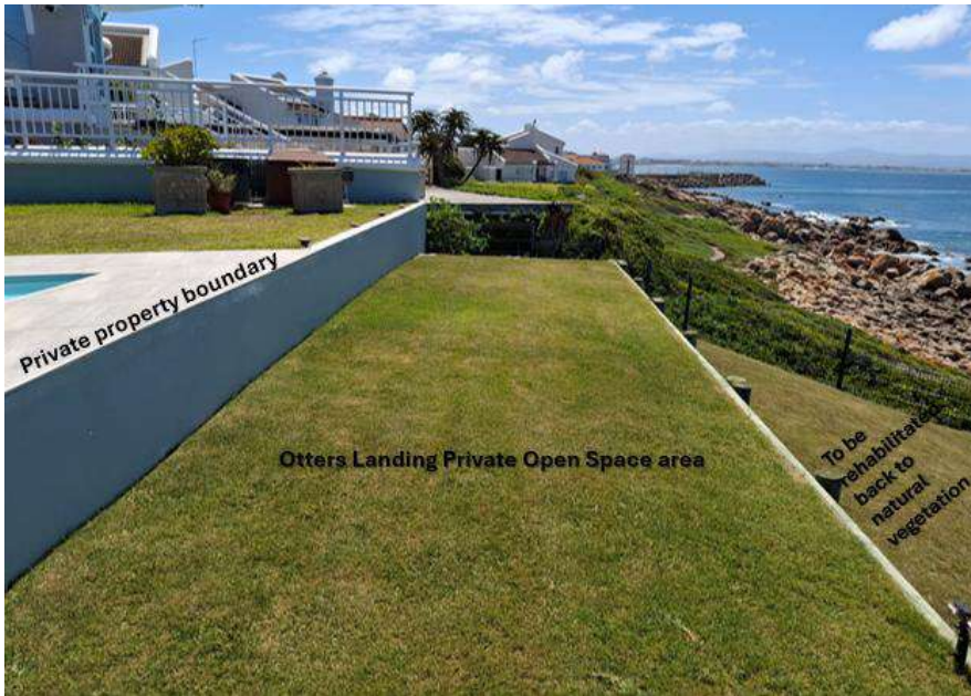
Figure 6: Terraced Garden for stabilized terrace embankment
